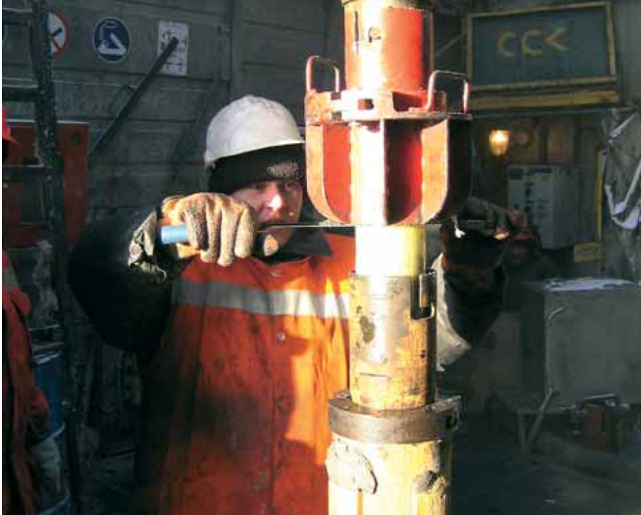
Coring in Progress
